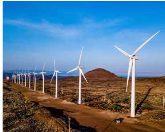
Lake Turkana Wind Power Project
